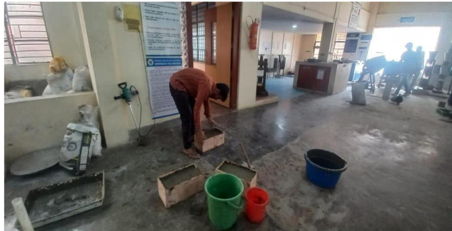
Casting of moulds
